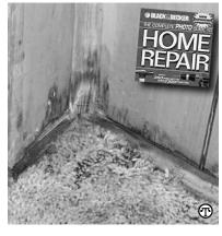
Repeated wettings have stained the paneling and carpet in this basement room. It is very likely that mold and mildew are growing in the carpeting and behind the paneling.
