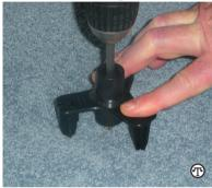
**Step three:** Place the gripper part of the fixture over the screw head. Then, rock the fixture left to right, until the screw head snaps off. The screw breaks at the weak spot that is consistently just below the surface of the floor.
