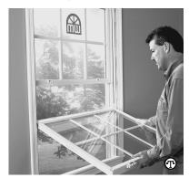
An easy-to-install sash replacement system can breathe new life into tired windows. The sash tilt in for cleaning and the system eliminates the need for storm windows.
