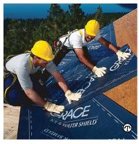
Using the proper roofing underlayment to repair damaged roofs also prevents future leaks.
