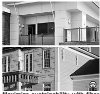
Maximize sustainability with fiber cement siding and weather barrier under siding.
