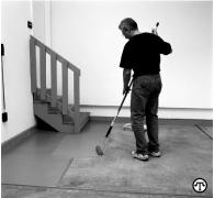
Epoxy coatings can revitalize and strengthen garage floors.
