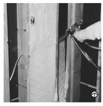
Installing an insulation/air barrier system can save you up to 50 percent in energy costs and help reduce a home's greenhouse gas emissions by thousands of pounds per year.
