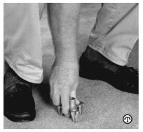
1) The first step in silencing a squeak is finding the joist. The kit comes with a tool designed for the job. Then, push the alignment and depth control fixture—also from the kit—into the carpet.
