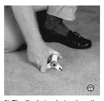
3) The final step is to place the gripper, which comes in the kit, over the head of the screw. Rock the screw until the head breaks off just below the surface of the floor, quieting the squeak.
