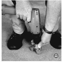
The next step is to place your weight around the fixture and drive the screw down into the floor as far as the fixture allows.
