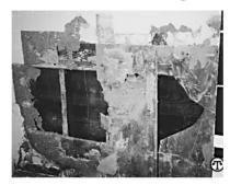
A little moisture seeping through grout does a wall's worth of damage when tile is attached directly to green board or plywood; experts recommend fiber-cement backerboards in kitchens and bathrooms.
