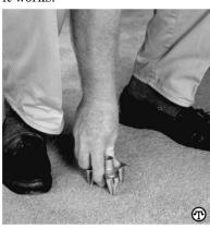
Step1: Locate the floor joist using the joist-finding tool in the kit. Push the Alignment and Depth Control Fixture firmly into the carpet.
