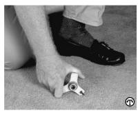
Step 3: Place the gripper part of the fixture over the screw head, then rock the fixture left and right, snapping the head off. The screw breaks at the weak spot that is consistently just below the surface of the floor.
