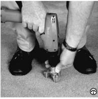
Step 2: Place your weight around the fixture and drive the scored screw down as far as the fixture will go.
