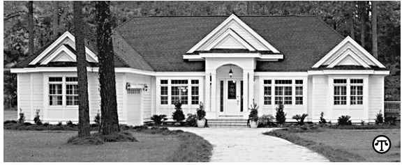
Homes such as the Bainbridge demonstrate the capabilities of off-site construction.
