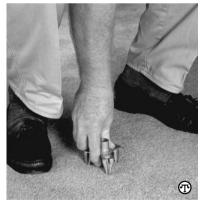
Step 1: FIND THE JOIST Locate the floor joist using the joist-finding tool provided in the kit. Then push the Alignment and Depth Control Fixture firmly into the carpet.
